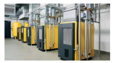
harness additional heat recovery by ducting exhaust air. In all, up to 96% of input energy can be recovered as heat.
