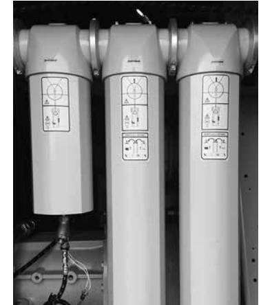
Water Separator and IQ Filters
